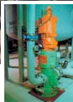
Feed pump for Isocyanate
