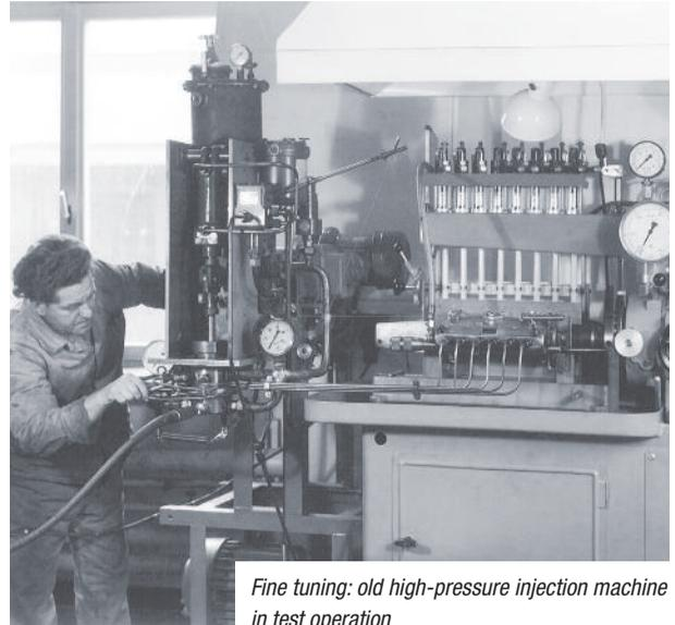
*Fine tuning: old high-pressure injection machine in test operation*
